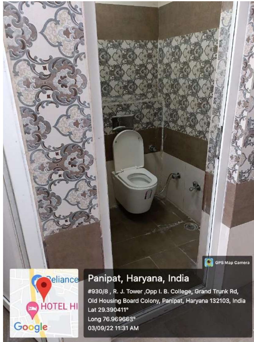
Figure 12 Differently Abled Friendly washrooms
