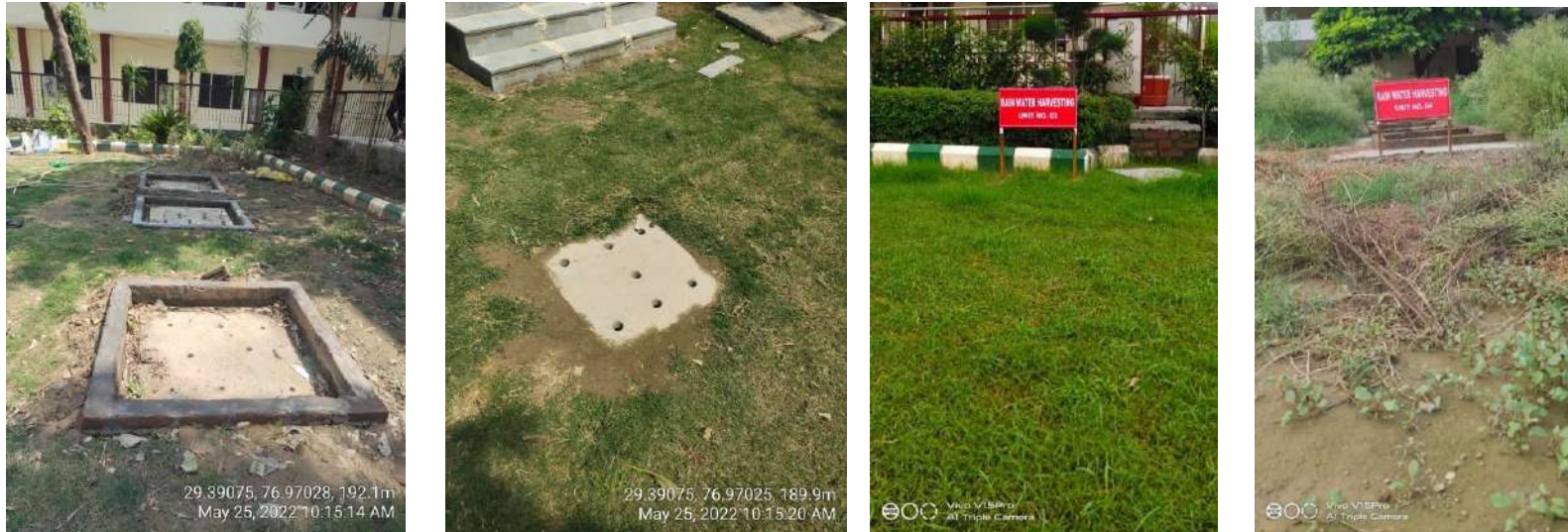
Figure 5 Rainwater Harvesting System
